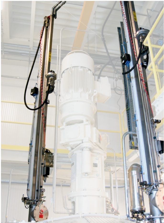
Lance system - moved and actuated pneumatically
